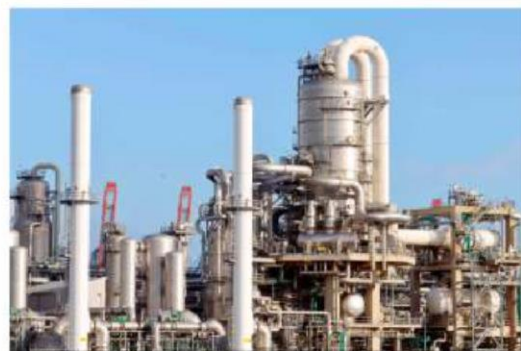
a structure for Application - Refineries
