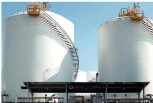
a structure for Application - Gas Storage
